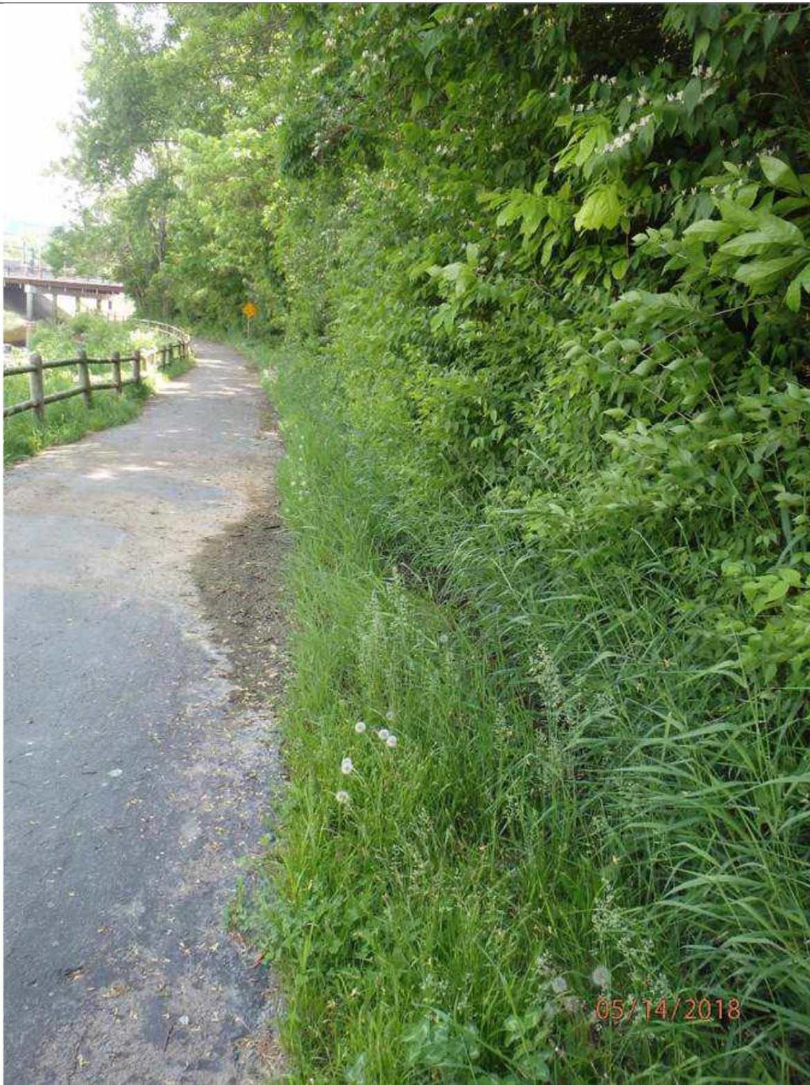
K – CUT DITCH - $7,150
