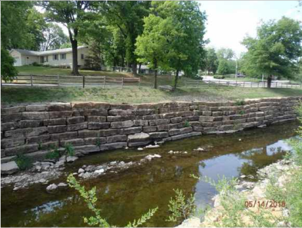
G – WALL REPAIR - $3,500
