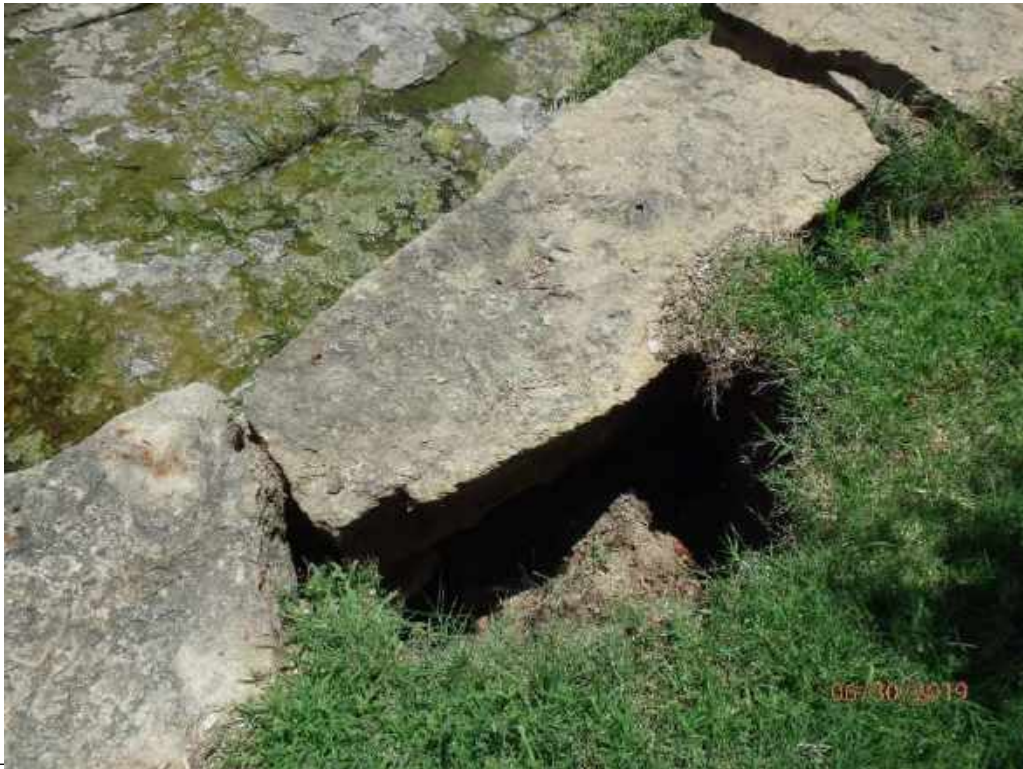
E – HOLE REPAIR - $500
