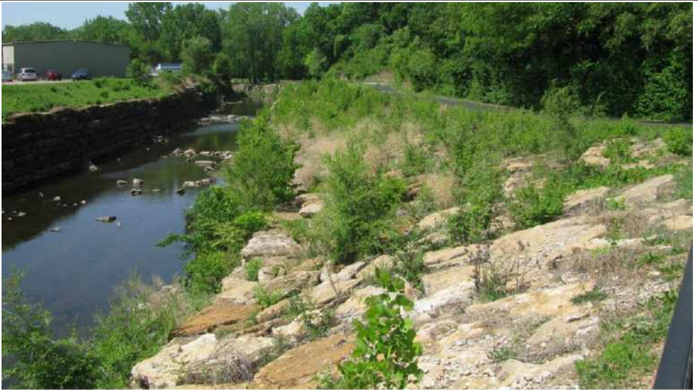
N – WEED AND FILL VOIDS - $4,000
