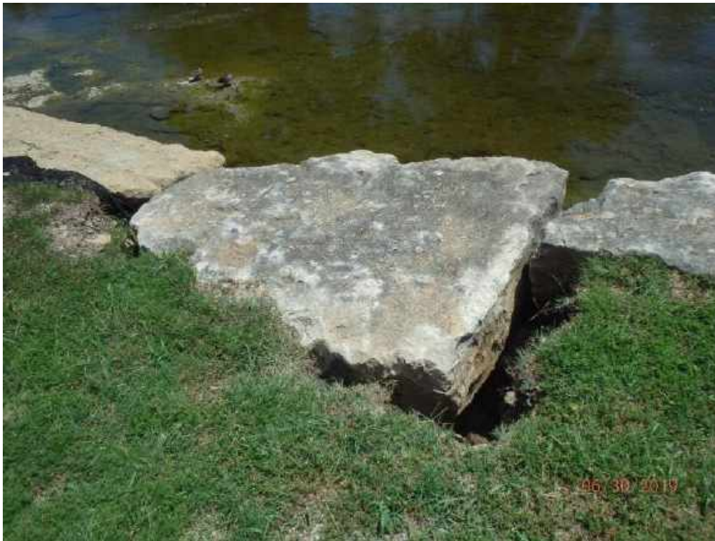
A – HOLE REPAIR - $500
