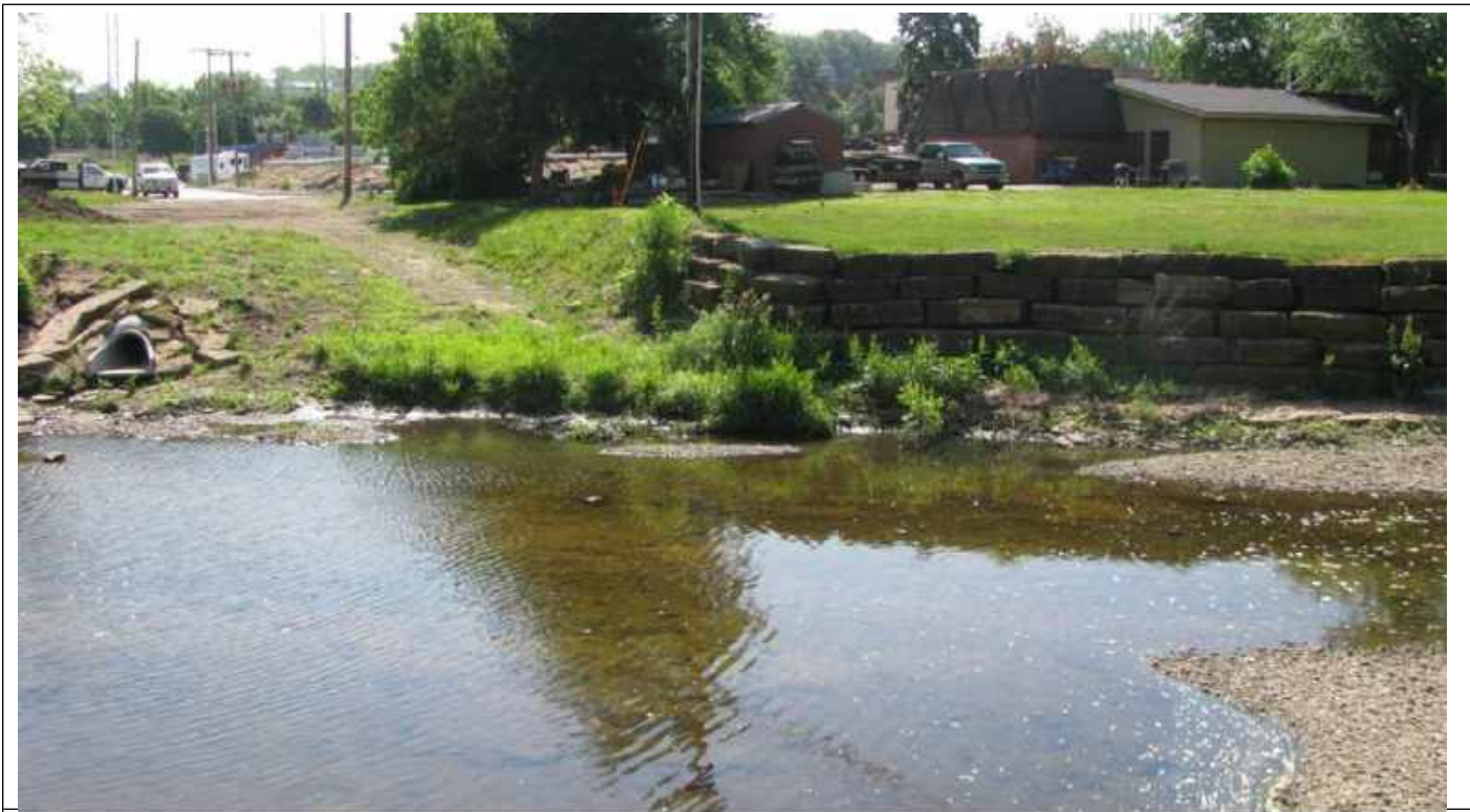
E – CONSTRUCT TOE WALL - $1,500
