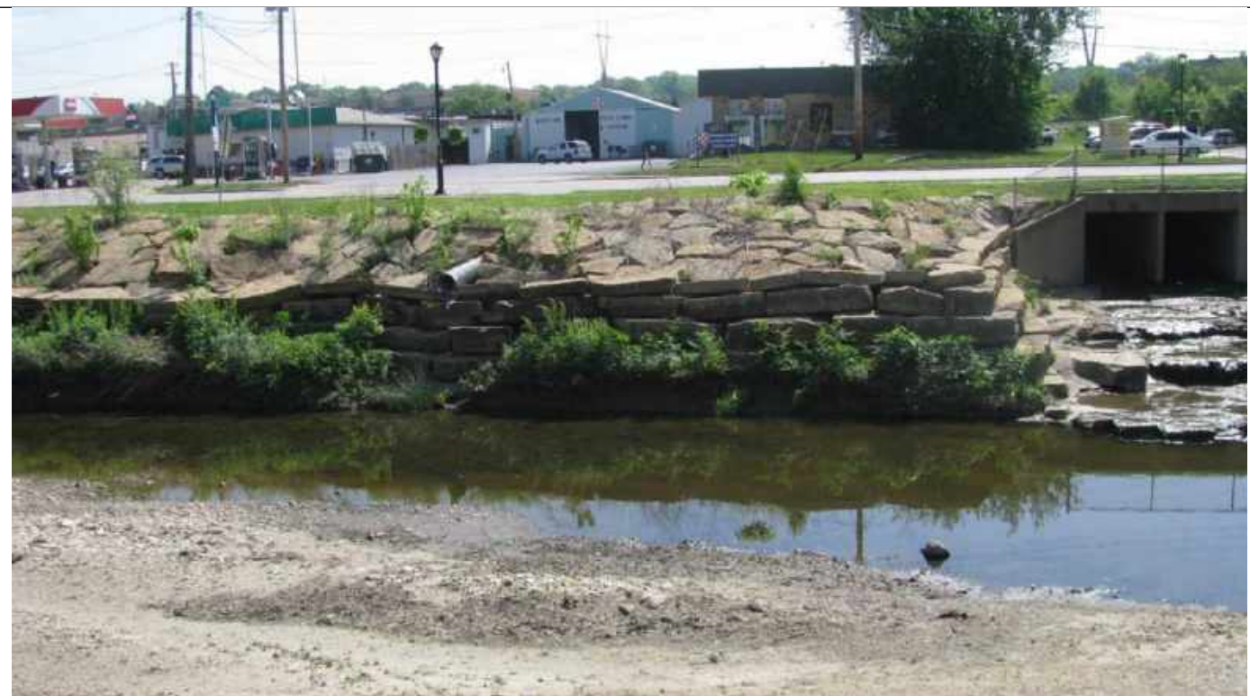
J – REBUILD WALL - $43,750
